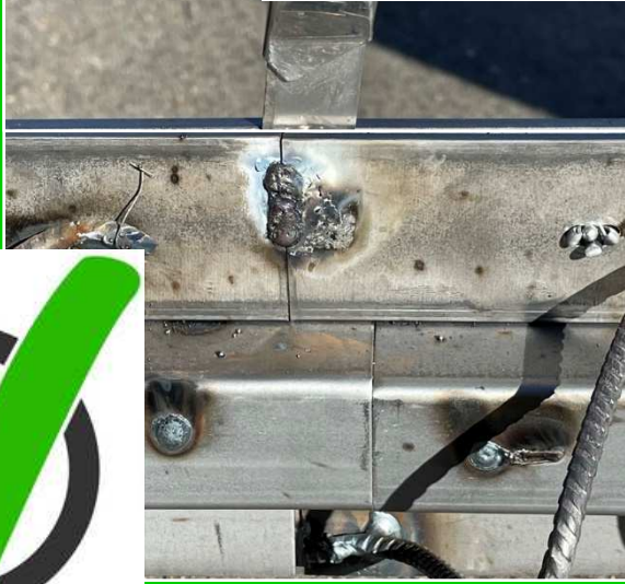
NO WELDING THROUGH THE TOP STRIP!
