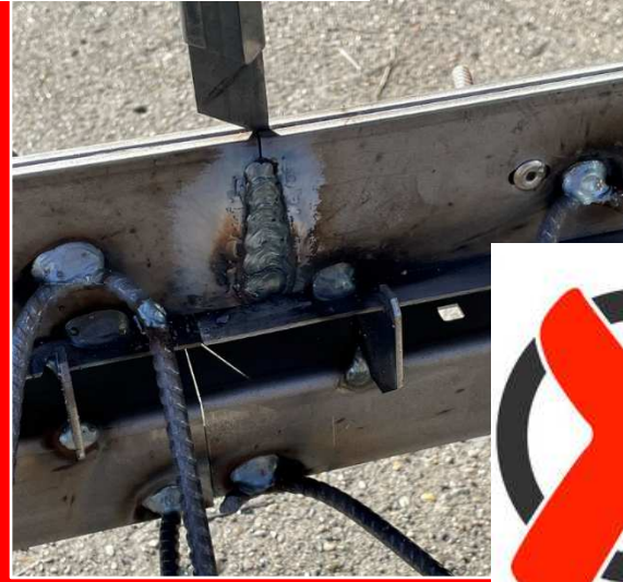
NO WELDING THROUGH THE TOP STRIP!
