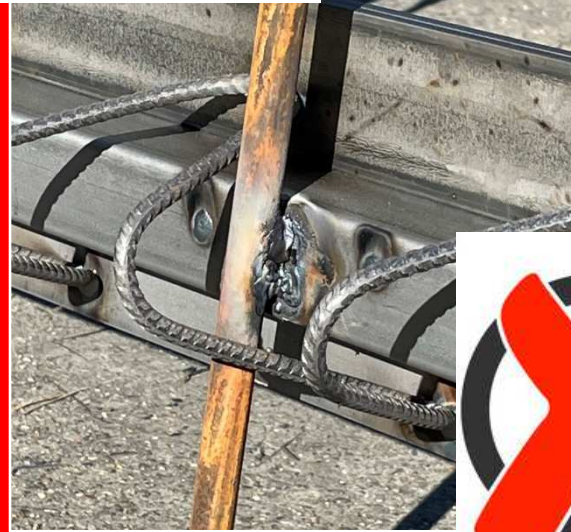
NO PINS WELDED AGAINST THE BODY!
