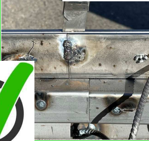
NO WELDING THROUGH THE TOP STRIP!
