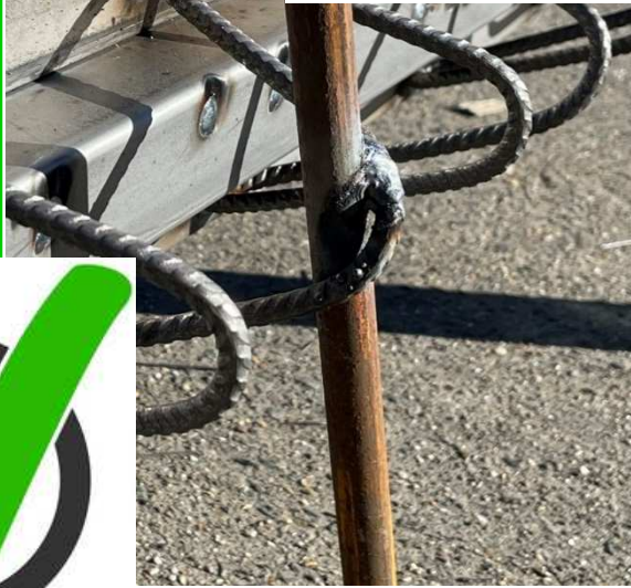
NO PINS WELDED AGAINST THE BODY!
