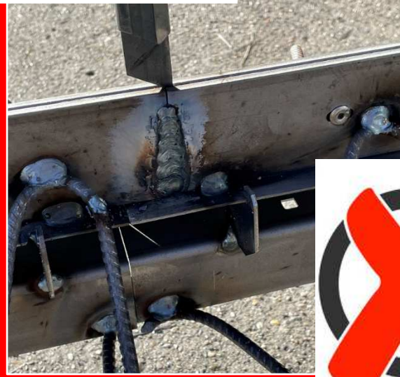
NO WELDING THROUGH THE TOP STRIP!
