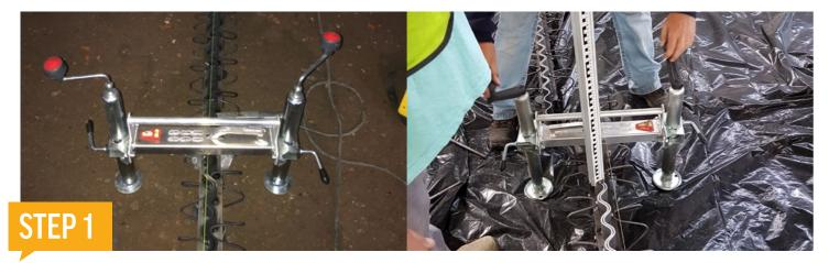
String a line in the location where the profiles are to be installed and lay the joints out along this line. Aligning is simplified if the line is not placed in the axis of the joint but on one side/edge of the upper sinus wave. Place the first joint parallel to this line and bring them to the correct height (using laser and the special developed adjustment tool). Check the vertical and horizontal level.
