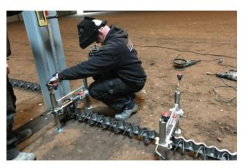
Place the next profile with its connection system in the first profile. See detailed instructions at the backside. With the connection, the start of this profile is immediately at the correct height. Bring the middle and the end of the second profile to the correct height with laser and adjustment tool. Repeat step 2 and 3 and weld the profiles together. Continue this way until arriving at an intersection, wall or column.
