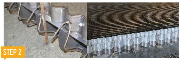
Hammer or drill pins (max. Ø 16 mm - 1/2 x 24" smooth dowels) into the ground vertically (slightly inclined in the direction of the joint longitudinal axis) inside the anchorage system with 2 on each side at the end of the profile. Two additional pins should be attached approximately in the middle of the profile (1 on each side) to ensure the correct position of the profile and to enable necessary adjustments.
