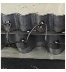
Check again the height level of the profile at the beginning, the middle and the end with a laser and also the horizontal and vertical level. Weld the pins to the profile. If welding work is not permitted on site, special adjustment feet are available. Pull down the falling steel plate to adjust the joint to the floor slab height. Adjustable feet pad shown in middle picture, which is recommended for slab on insulation, topping slabs and other installations.
