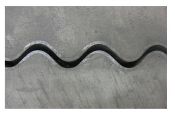
To become a satisfied result of the sinus slide® jointing solution, it is absolutely necessary to finish carefully the concrete at the same level as the sinus joint edges. SEE BACK SIDE OF THIS GUIDELINE.
